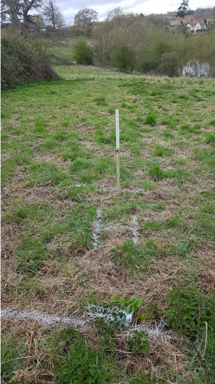
HG8 – view over the existing fence towards the proposed boundary (peg and white line) with the white line (foreground) marking the edge of the proposed track and the proposed 2m wide hedge and trees (painted 'H') in between.
