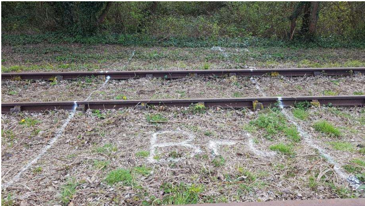
TB12 – view looking south from the white painted cross of the approximate location of the bridge.
