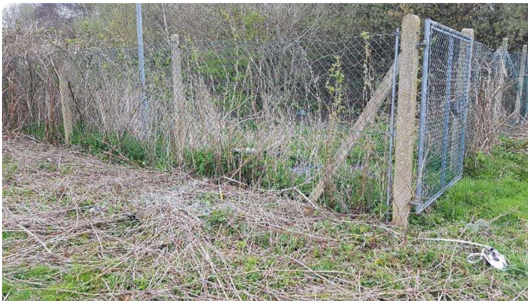
CR2 – end of tape marks position of proposed ramp.
