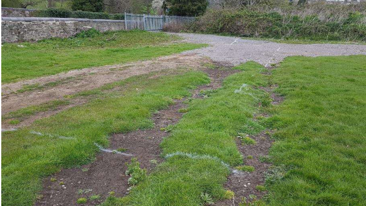
CR9 – Proposed permanent boundary in the foreground looking towards new gate, with dashed line marking edge of surfaced area heading towards the top of the photo.
