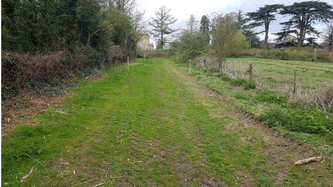
HG13 – view up towards Chapel Pill Lane. Pegs mark the width of track with grass verge to existing hedge on the left and proposed hedge on the right in the view.
