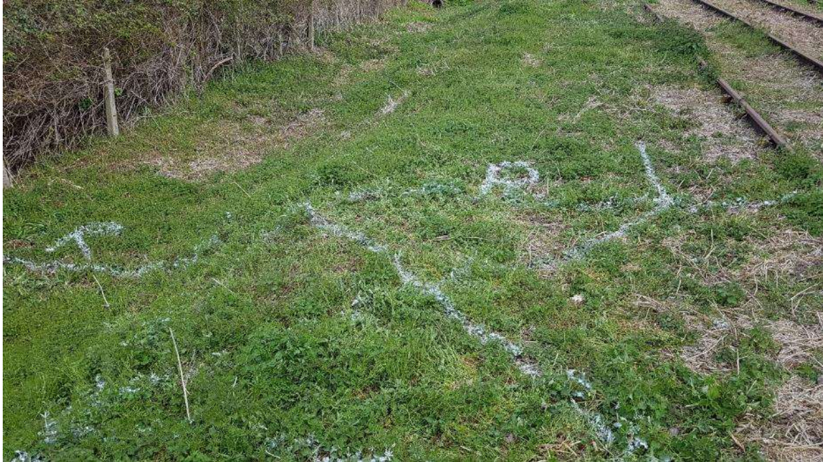
TB11 – top and bottom of ramp, and the white paint cross marks the landing between the top of the ramp (R) and the bridge which is off to the right of view.
