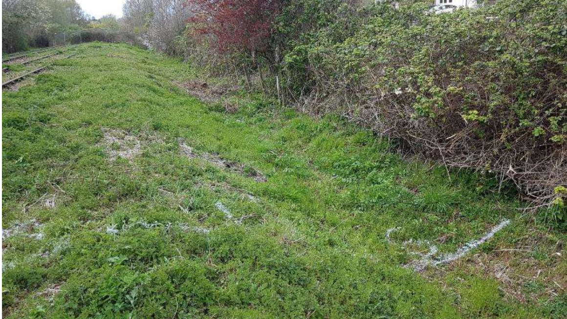
TB9 – white paint marks the top and bottom of the steps (S) with the peg in background marking the corner return (TB8)
