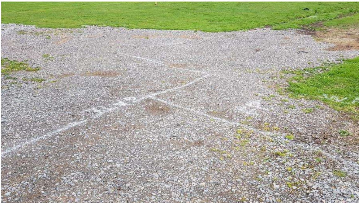
CR10 – view of gate (GATE on ground), footpath (FP) and wall (WALL) meeting point. Dashed line off top right marking edge of surfaced area.
