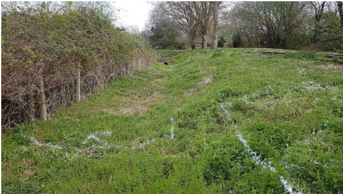
TB10 – Bottom (left) of the ramp (R) which crosses the existing path at TB6 and returning at TB5 (see above) with top of ramp (right).
