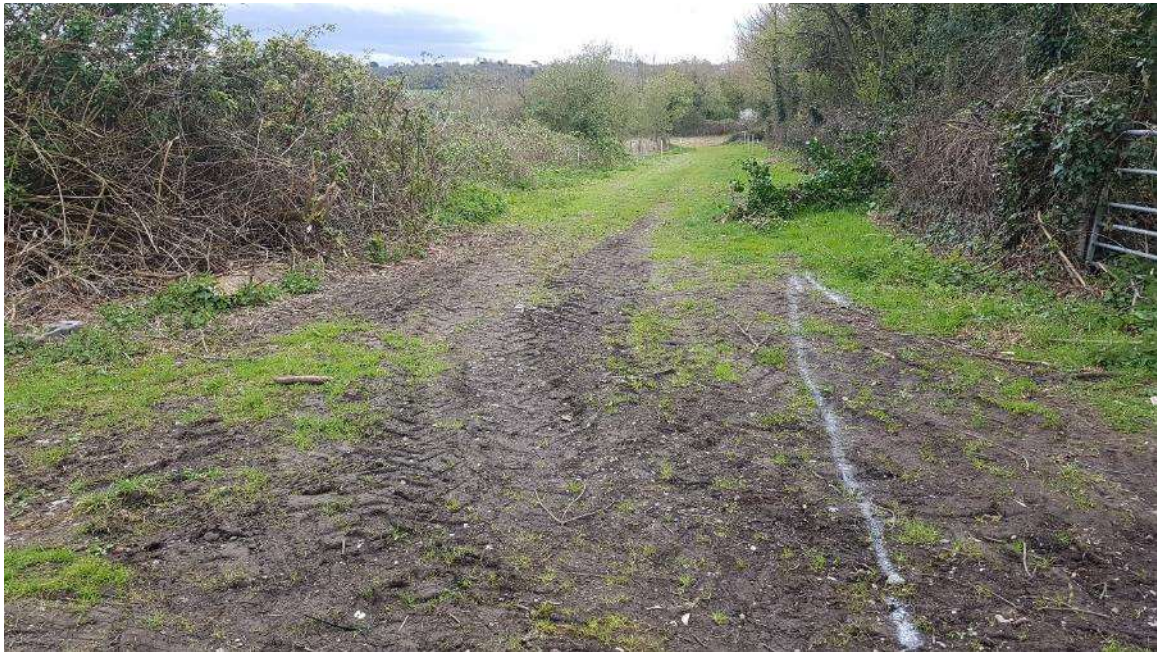
HG14 – view down the track, white line is the proposed track edge with existing gate on right replaced by new boundary fence.
